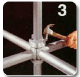
Tighten with a hammer blow
